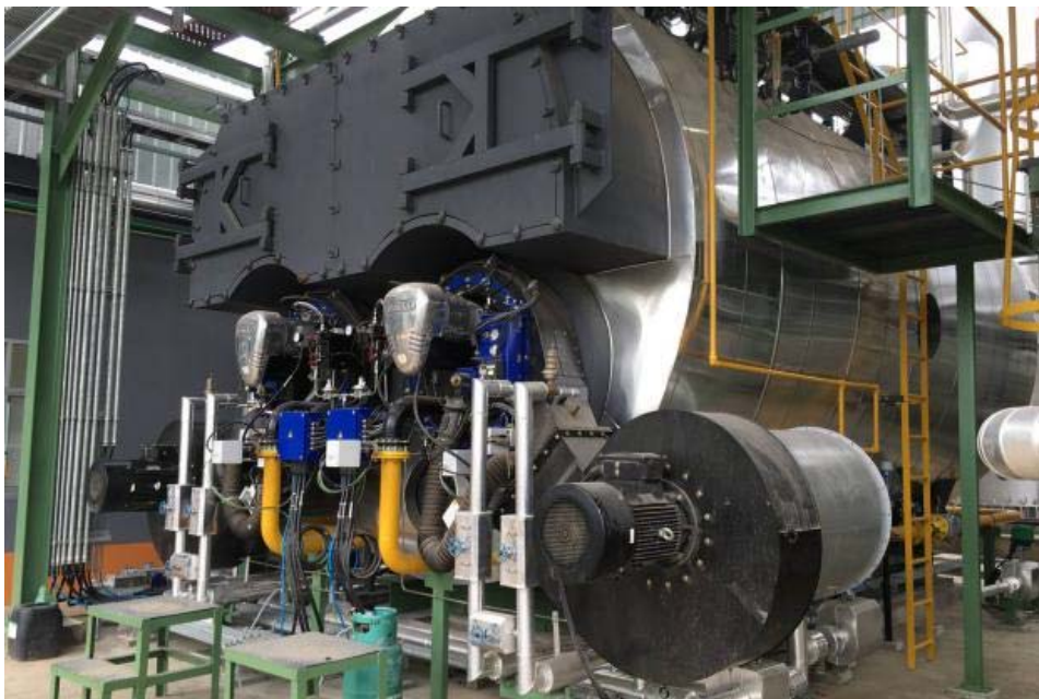
GETABEC DOUBLE FLAME TUBE BOILER
